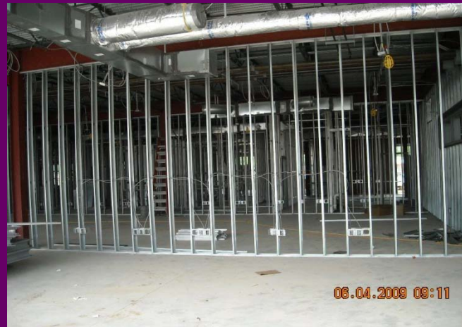
Interior walls being installed in the 6 th and 7 th Grade Academic
