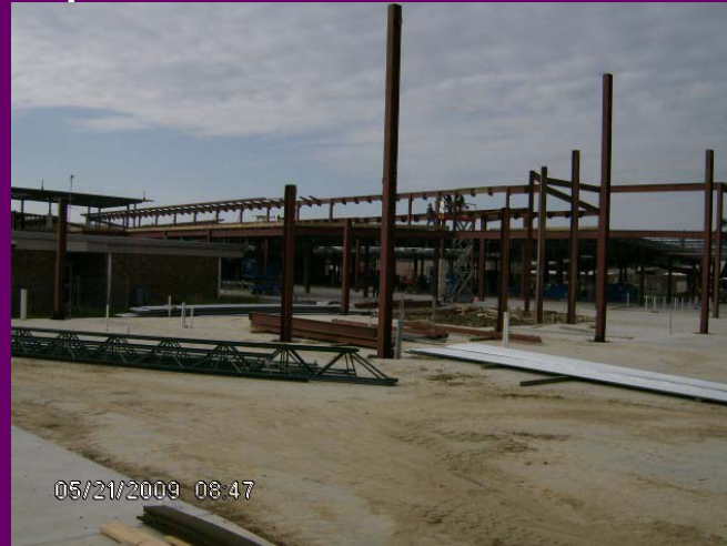
Structural steel being erected at the CATE building
