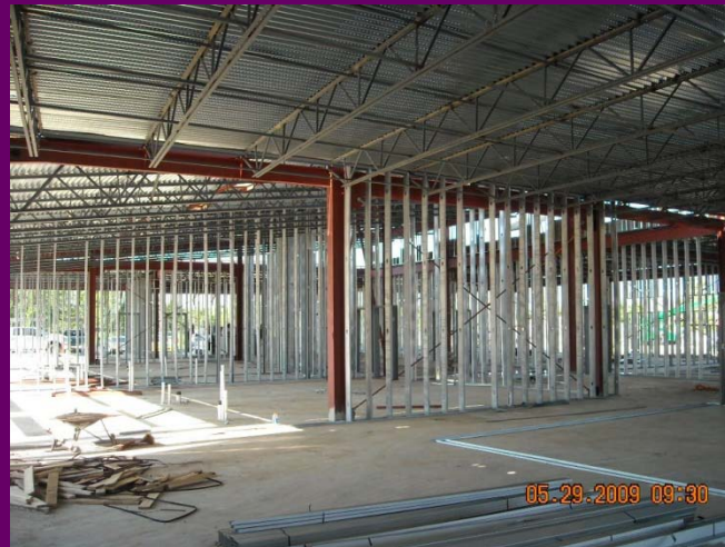
Interior walls being installed in the Academic Wings
