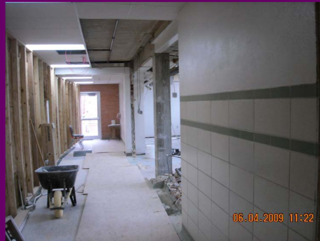
Demolition work has started in the connector area
