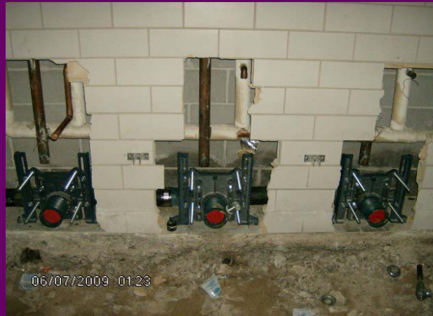
New toilet carriers being installed in the restrooms at Taft Elementary
