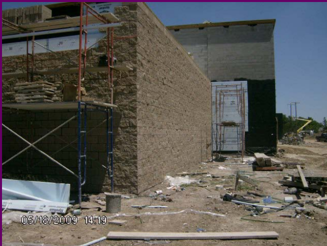
Face block being installed on the Gymnasiums
