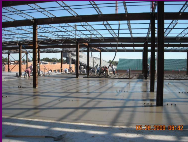
Concrete slab placement on the 2 nd level is complete
