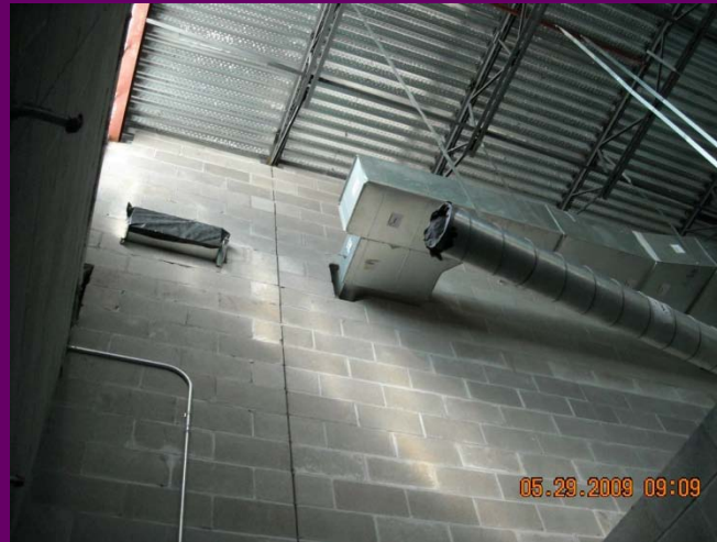
HVAC duct work being installed in the Gymnasiums
