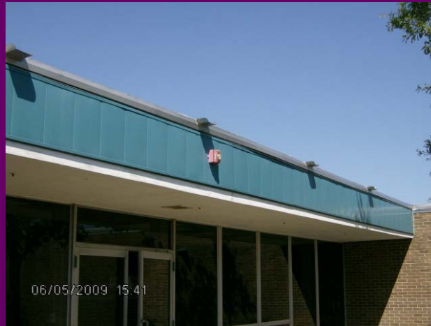
Scuppers on the roof at Taft Elementary
