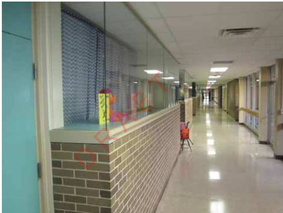
PHOTO TES4 - CORRIDOR/CLASSROOM WALLS
