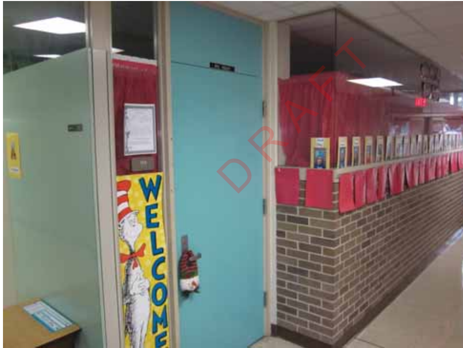
PHOTO TES5 - CORRIDOR/CLASSROOM WALL AND DOOR
