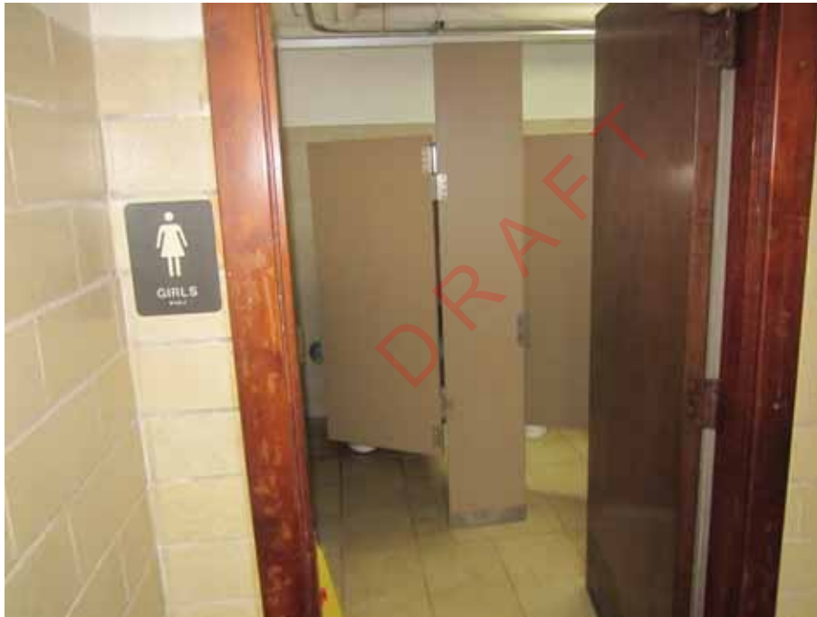
PHOTO GES3 - GANG RESTROOM
