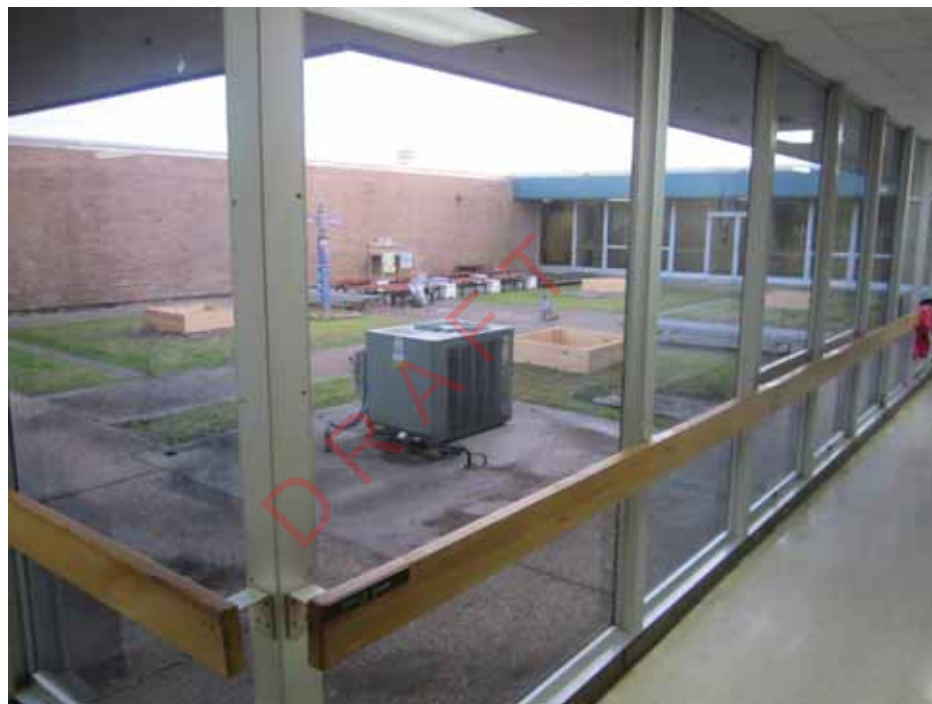
PHOTO TES6 - COURTYARD
